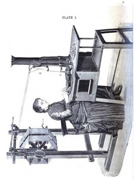
Cocoon-reeling machine simplified and arranged for cottage use.
